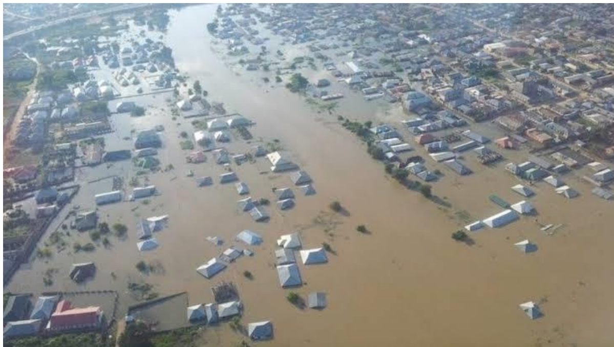
Fig 5: Aerial view of flooded areas in Nigeria as at 2022 (the cable, 2022).
