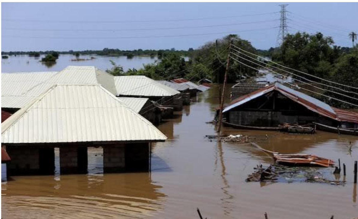
Fig 4: A destroyed home/village during the 2022 Nigerian Flood (the globe and mail, 2022).
