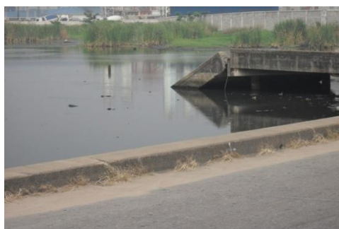
Plate 12. Collapsed bridge at the National Theatre, Iganmu, Lagos Source: Obiadi (May 14, 2011).
