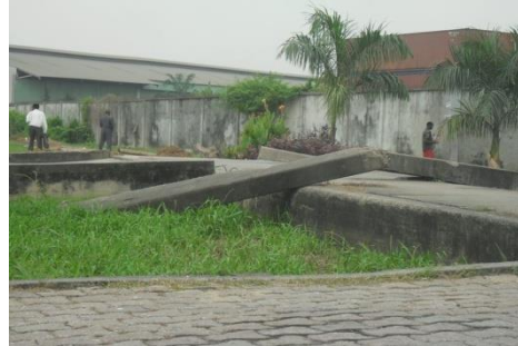
Plate 14. Collapsed pedestrian bridge at the National Theatre, Iganmu, Lagos Source: Obiadi (May 14, 2011).
