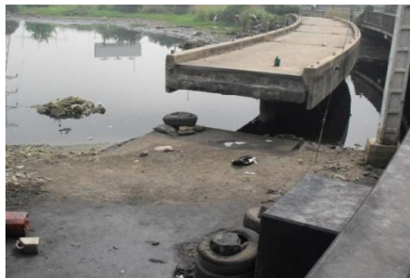
Plate 9. Collapsed bridge at the National Theatre, Iganmu, Lagos Source: Obiadi (May 14, 2011).
