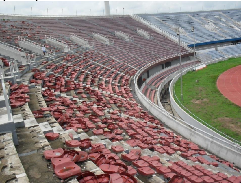
Plate 3. Collapsing seats at the National Stadium, Sulurere, Lagos Source: Obiadi (May 25, 2011)
