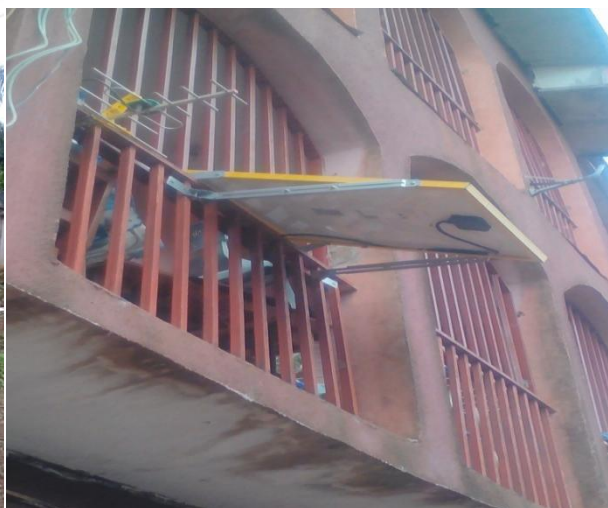
Mobile Telecommunications Network (MTN) Solar Home system at a residential building
